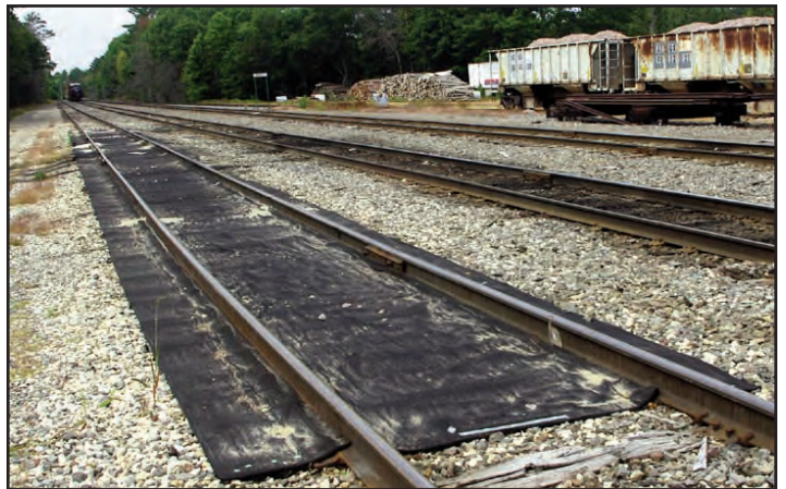
Track mat at the flange oiler at Dixon Illinois on the UP.
