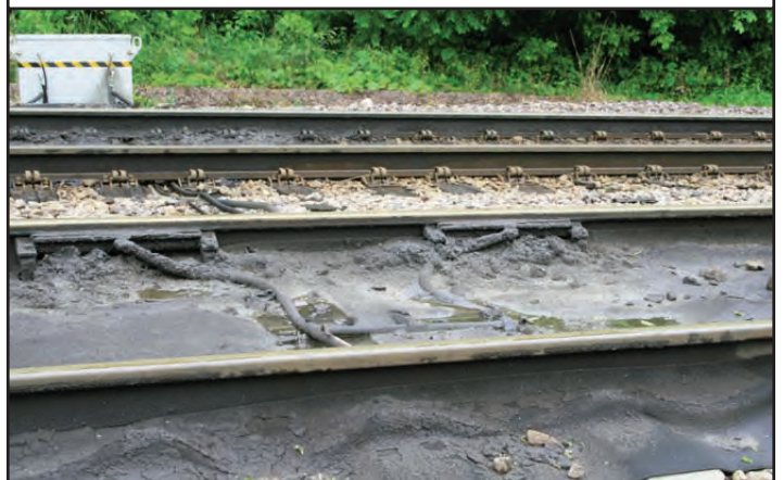
Track mat at the flange oiler at Dixon Illinois on the UP.
