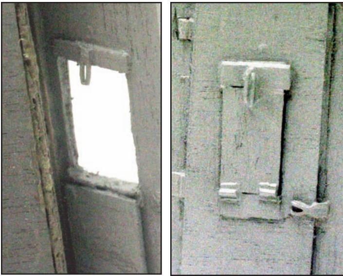
Detail of the opening on the operator's cabin and the door.
