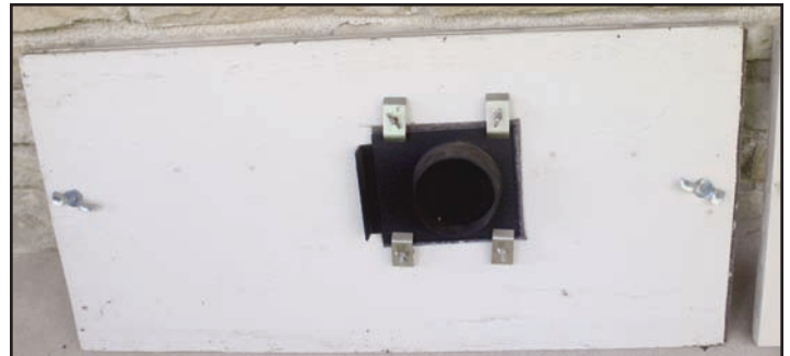
Photo of the window vent.
