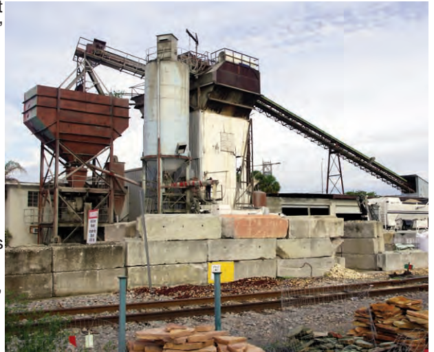
Another photo of the concrete plant. More on page 10. All photos by David Leider.
