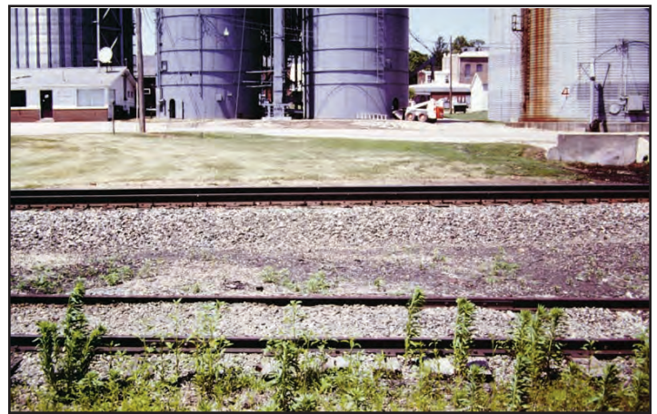
Sidings are lower than the main. Elmwood, IL on the Burlington Northern.
