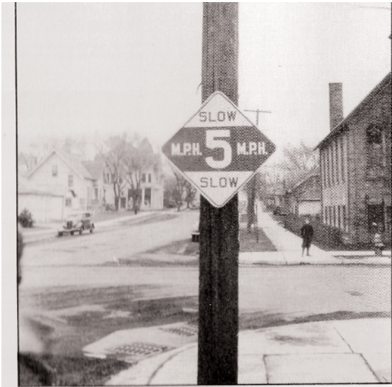
Standardized Type of Slow Sign with Indicated Allowed Speeds of 5-10-15 M.P.H.
