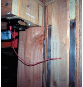
Figure A -micro switch at swing gate
