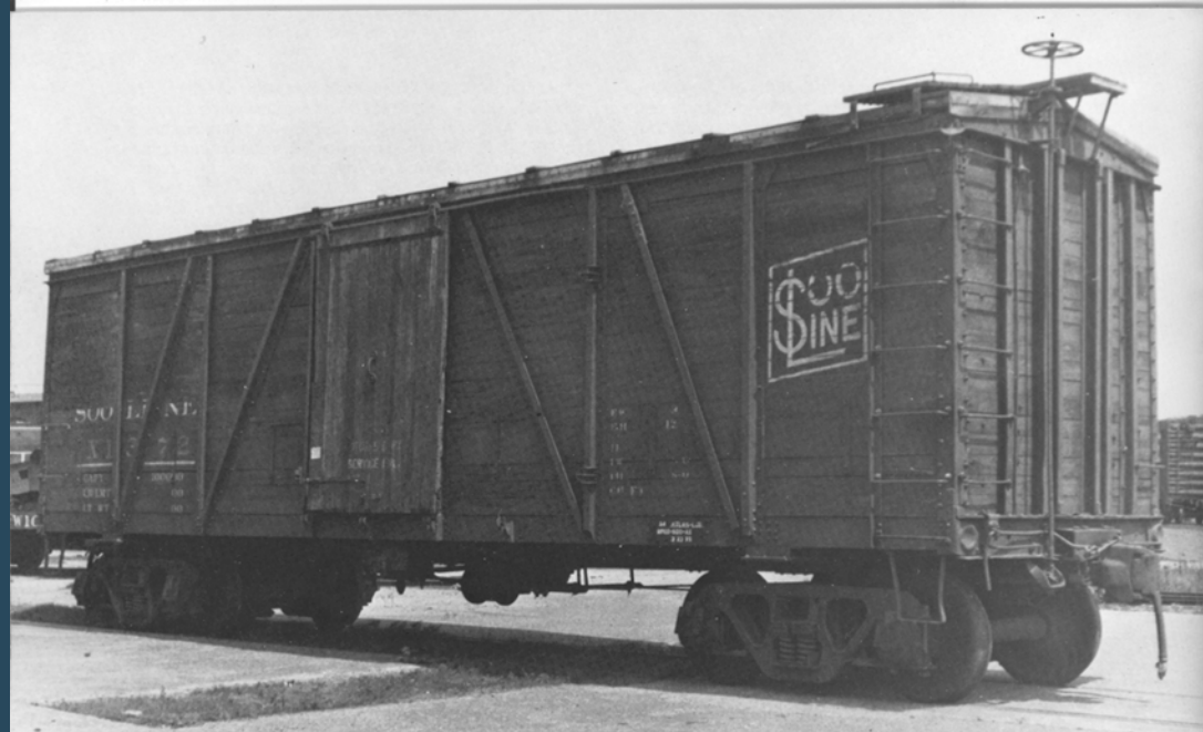
Car X1372 was built as Soo Line 13516 in 1912. It is an example of a Type 1 boxcar, being a member of the first series of outside braced boxcars cars built for the Soo Line. Here it is shown in work equipment service as a Stores Department car used in moving company supplies. The car was retired in February, 1981 and sold to Interprovincial Steel in Regina for scrap in April, 1981. The photo was taken in June, 1980 at Shoreham by Stu Nelson.
